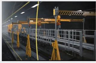
3. Remote controlled chain hoists lift new rail or switches into the worksite. The hoist is then used to exchange the Rail or switch
