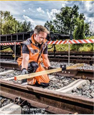
Measuring device for frog nose incline Grooved rail adjustment Check rail level measuring device Transport bag for segmented devices Transport and storage case
