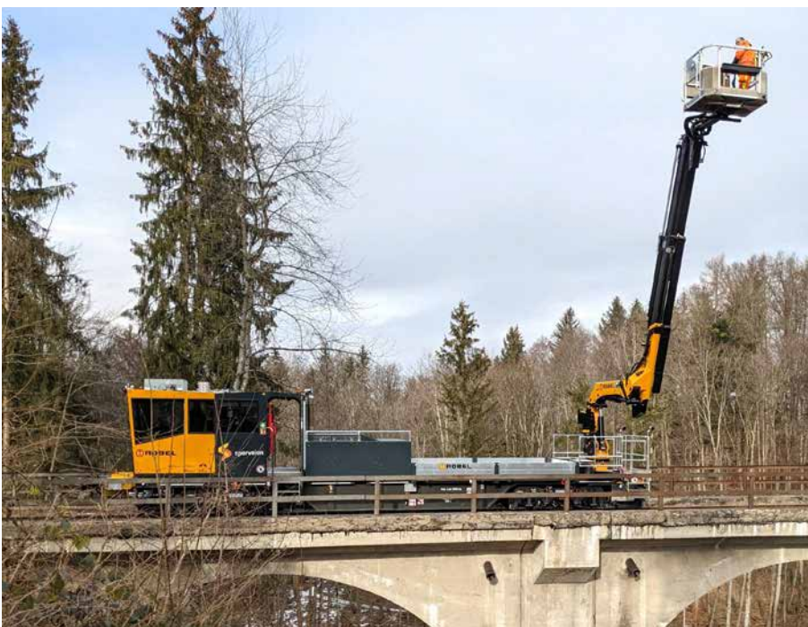
Fig. 7: Robel uses the Chiemgauer Lokalbahn line (here: Ameranger Viaduct) for testing and measuring runs in preparation for dynamic commissioning and authorization.
