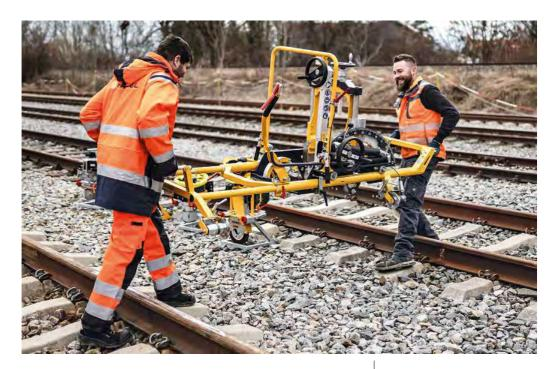
Easy to handle: the ROGRIND 13.63 modular rail and switch grinding machine can be mounted with additional modules on a base frame that can travel on rails.
