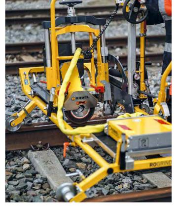
Environmentally friendly: the ROGRIND 13.63 can also be operated without emissions using energy from the battery storage.
