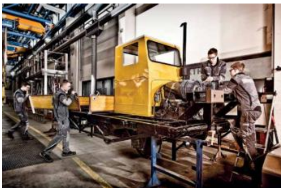
Within four years, 22 apprentices reconditioned this Robel crew car from the 1950s.
