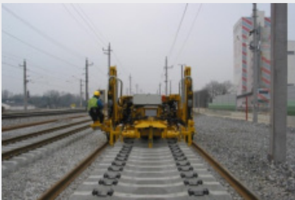
Lay sleepers accurately and evenly, ready for rail installation
