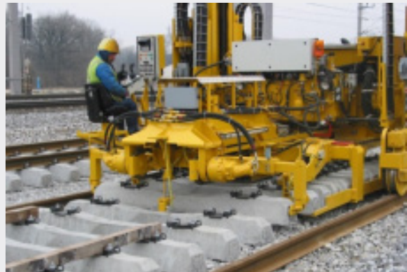
Sleeper placement tolerance to the nearest millimeter – approx. 5 sec. / sleeper
