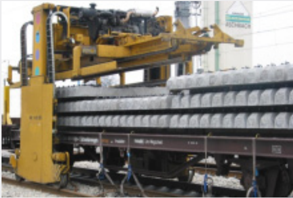
Lift up to 20 concrete sleepers from the trolley
